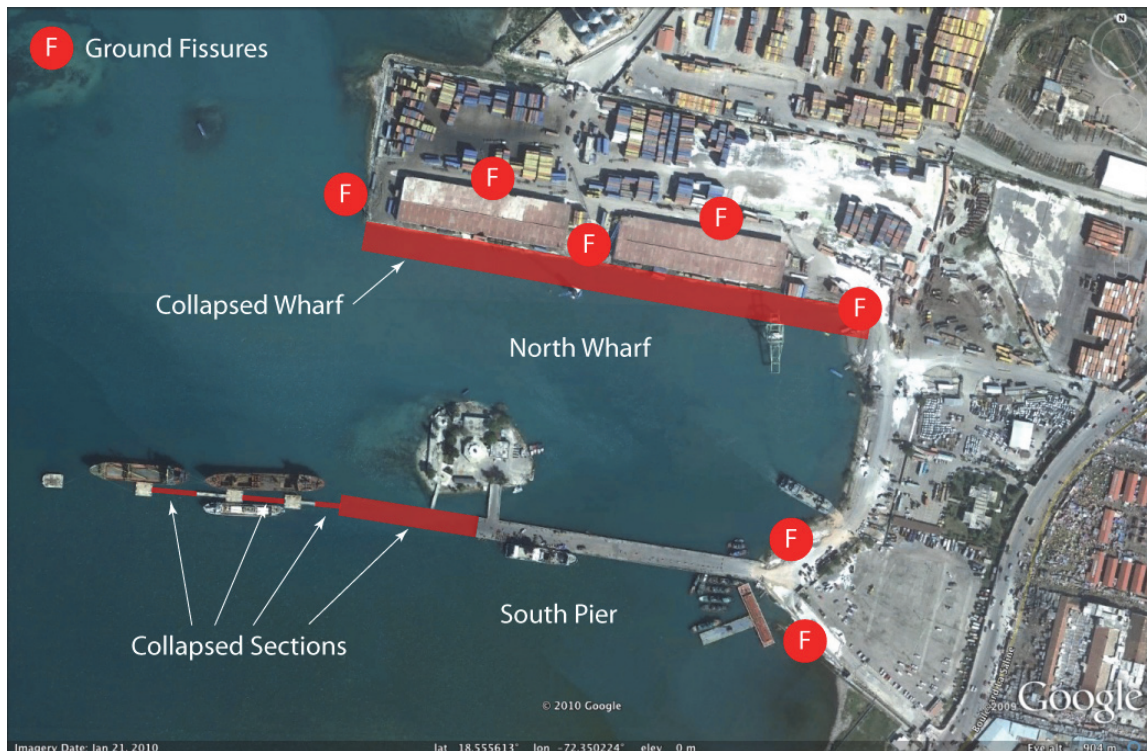
Figure 2-2 Annotated aerial Google Earth image of Port de Port-au-Prince showing the impacts of the 2010 Haiti earthquake. Circles with embedded “F” denote locations of ground fissures. Light-colored areas depict locations where sand boils occurred.
